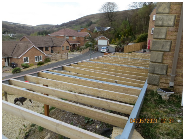
Fig. 1.6 View from decking
